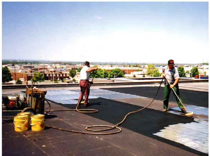
*Hi-Tuff adhered to substrate with bonding adhesive.*
