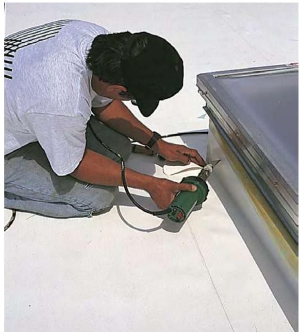
*Corner fabrication with a hot-air hand welder.*
