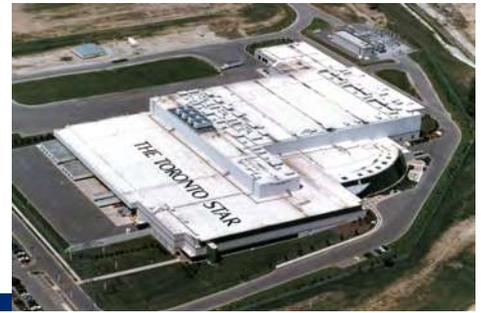
damage occur, it can be easily found and quickly repaired. Aging has virtually no effect on the membrane's 'weldability' so it can be as easily repaired five years from now as the day it was put on.
